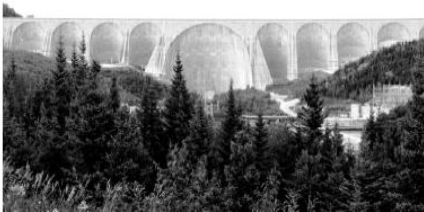
DANIEL JOHNSON DAM (CANADA, 1968, 214 m height)
